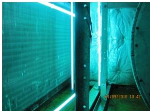
Coils and drain pan in AHU-3 before and after bathed in very high output 253.7 nanometer Germicidal UVC Light
