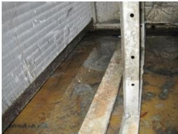
Coils and drain pan in AHU-3 before and after bathed in very high output 253.7 nanometer Germicidal UVC Light
