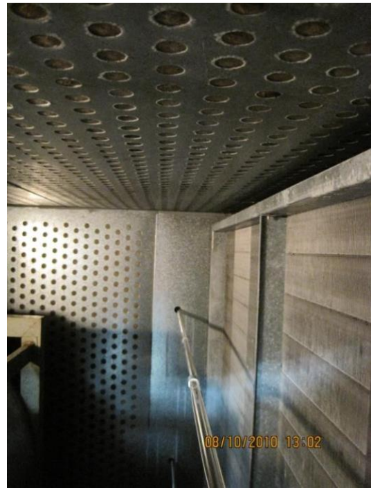
AHU T2-20 plenum with Steril-Aire very high output UVC Emitters™ installed
